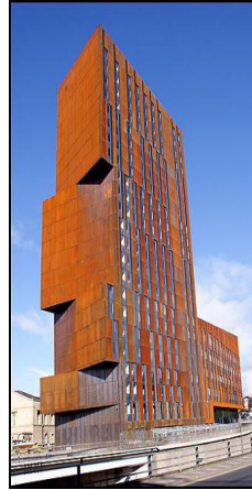
Resim 1. Broadcasting Tower, USA (URL.1)
